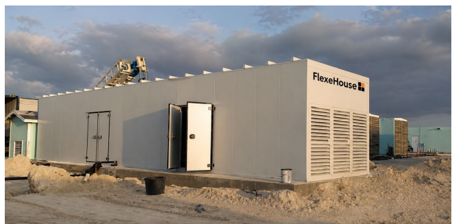
On site — louvred ventilation and access doors deployed in desert conditions.
